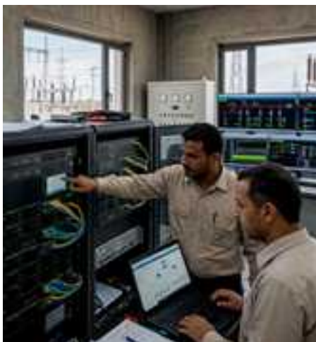
Substation Automation Project
