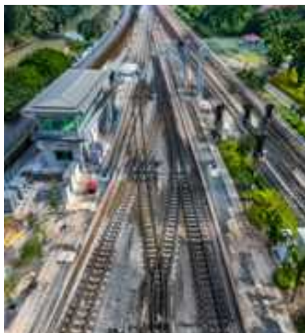
Thailand Railway Signal Control Project
